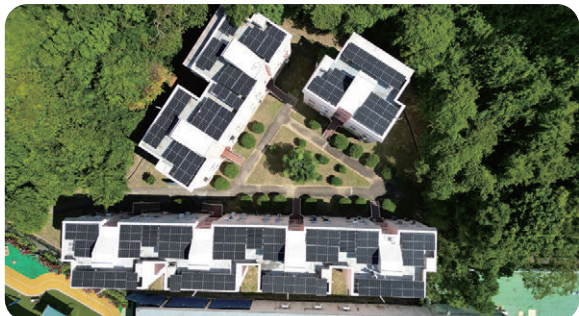
Solar Panels at Staff Quarter
